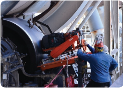
Support roller grinding with electronic circumferential measurement
