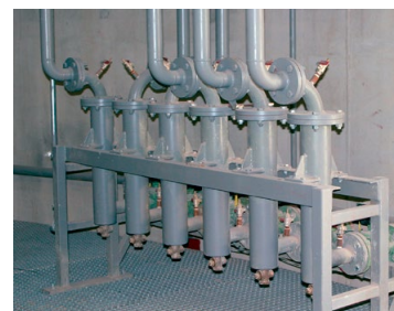
Figure 6: Filter battery for a single tank outlet (optional)
