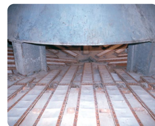
Figure 3: Steel cone to relieve pressure above outlet
