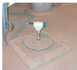
Manhole and nivopilot on top of the silo
