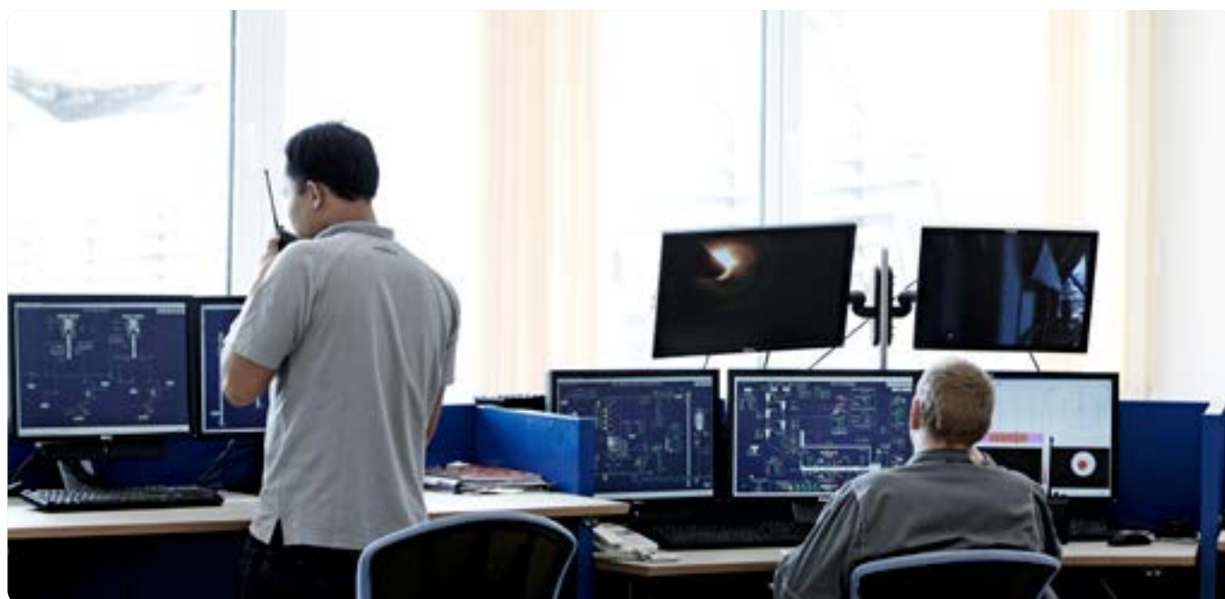
ECS Control Center
