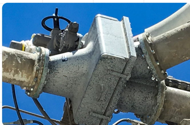
SK V2 2-way diverter valve
