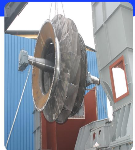
Impeller, delivered pre-assembled
