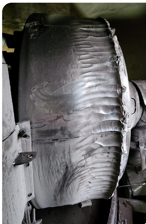
Severe uneven roller wear.
