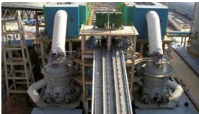
Twin mill installation
