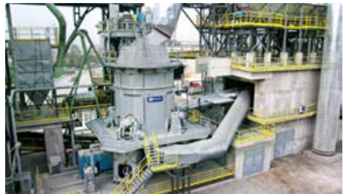
OK™ mill installation
